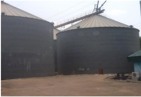
Storage Facility for CGI
